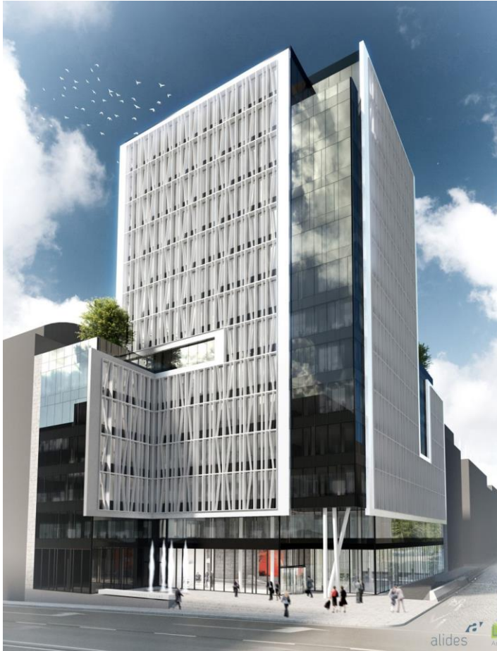
Immeuble Alides, LD2, 2018
